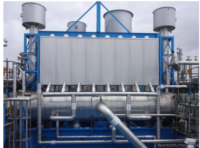
Figure 8: insulated HP drum with DrumPlus-technology at El Segundo CCPP, California USA.
