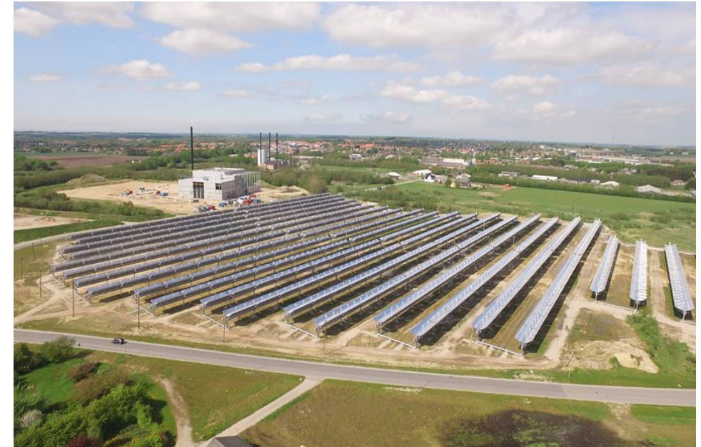
Hybrid CSP + Biomass Boiler + ORC for a District Heating scheme in Denmark (photo courtesy of Turboden S.p.A.)
